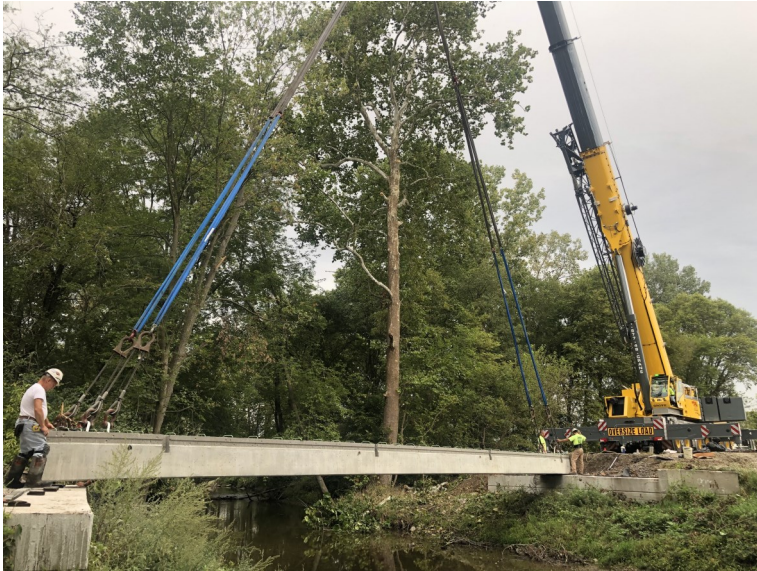
R&I Construction working on BR TR 209-0.18
